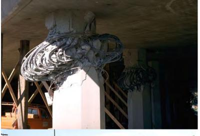
Steel-reinforced concrete support beams damaged by the 1994 earthquake
